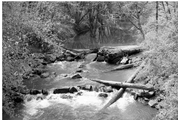
A boulder log stream structure in the upper Siuslaw
