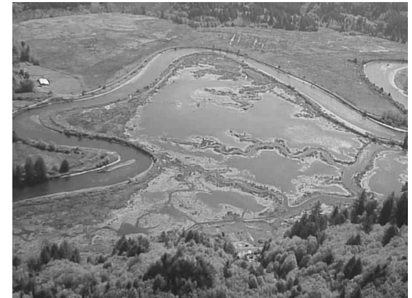
A dike breach at the North Fork
